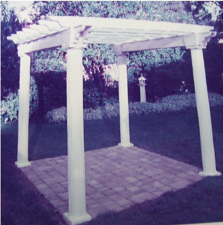
Rick's Garden Structure, note the curved ends which was done on a CNC. Phil Shannon demonstrating the Drill Doctor. The Drill Doctor and the collet used to hold the drill bit. Another attachment for grinding drill bits and some large drill inserts brought in by Brian.
