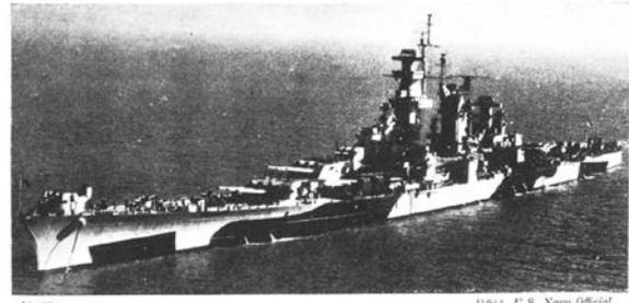
At full scale she is 808'6" long and displaced over 34,000 tons loaded for combat. Powered by four steam turbines, top speed was 38mph, cruise range was 14,000 miles, and she even carried catapult-launched seaplanes: there *must* have been a very cool machine shop somewhere inside her hull!
